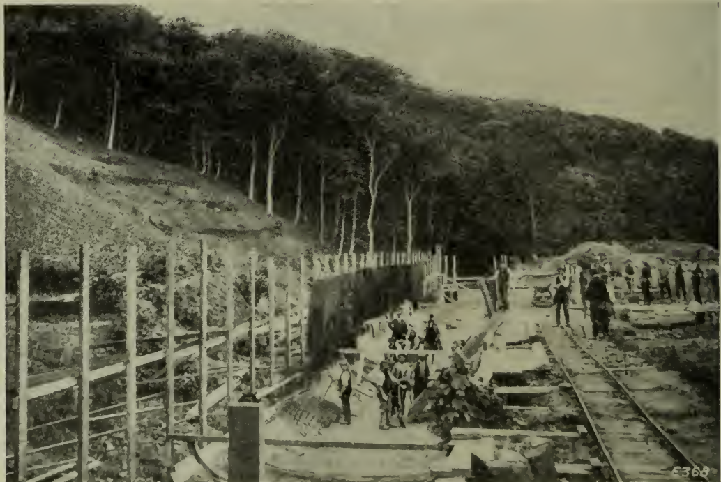
REINFORCED CONCRETE CULVERT IN COURSE OF CONSTRUCTION AT CRIMDON DENE.
